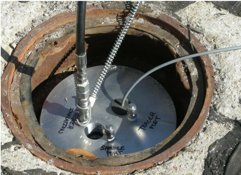
Figure 1.2-3 Surface completion for borehole 54-24399.
